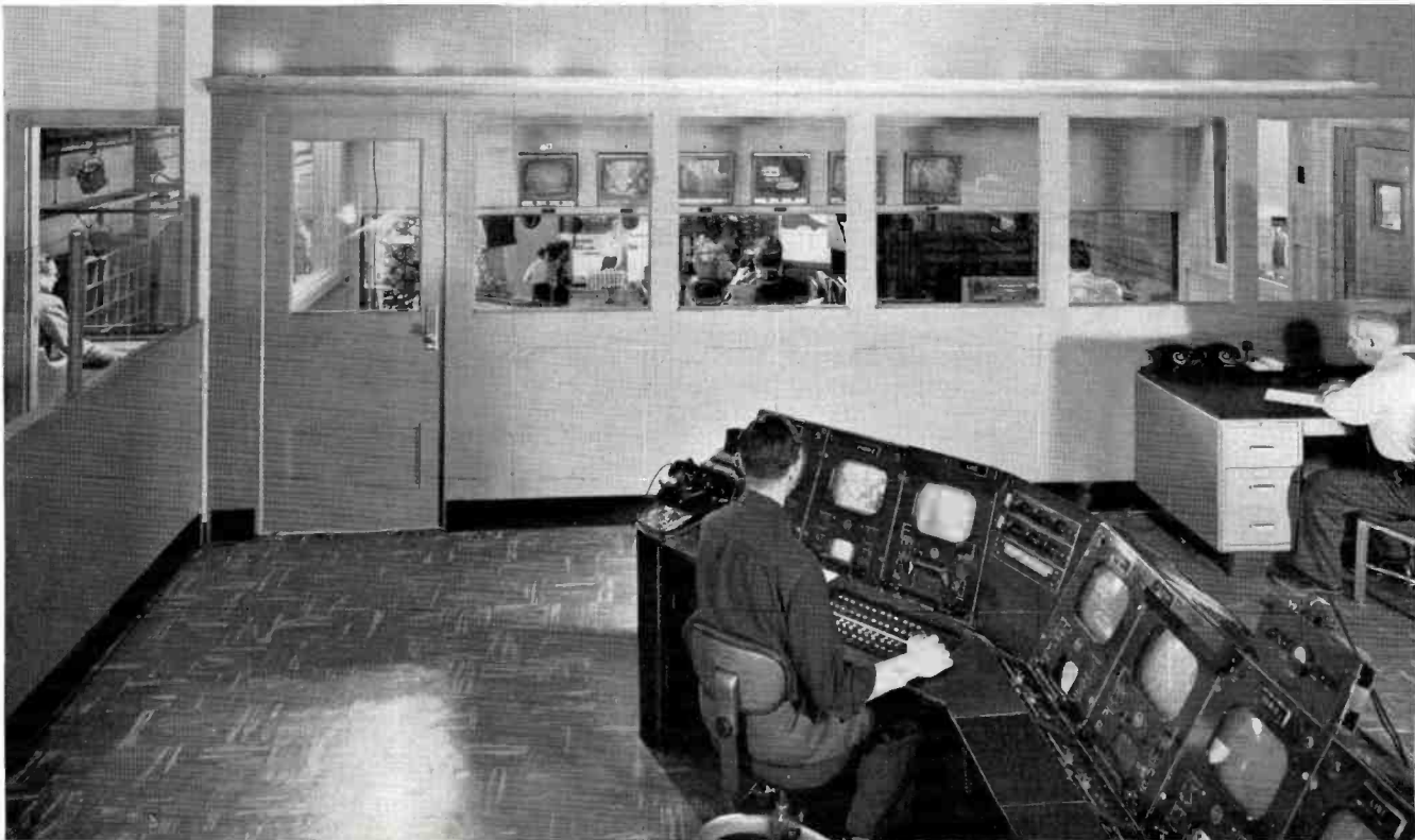
FIG. 7. View from the TV master control room through the director's booth into the studio. Director and audio operator (in booth) have an unobstructed view of studio, see camera pictures on monitors mounted in wall above studio window. Announcer's booth is at extreme right; clients' booth at far left.
