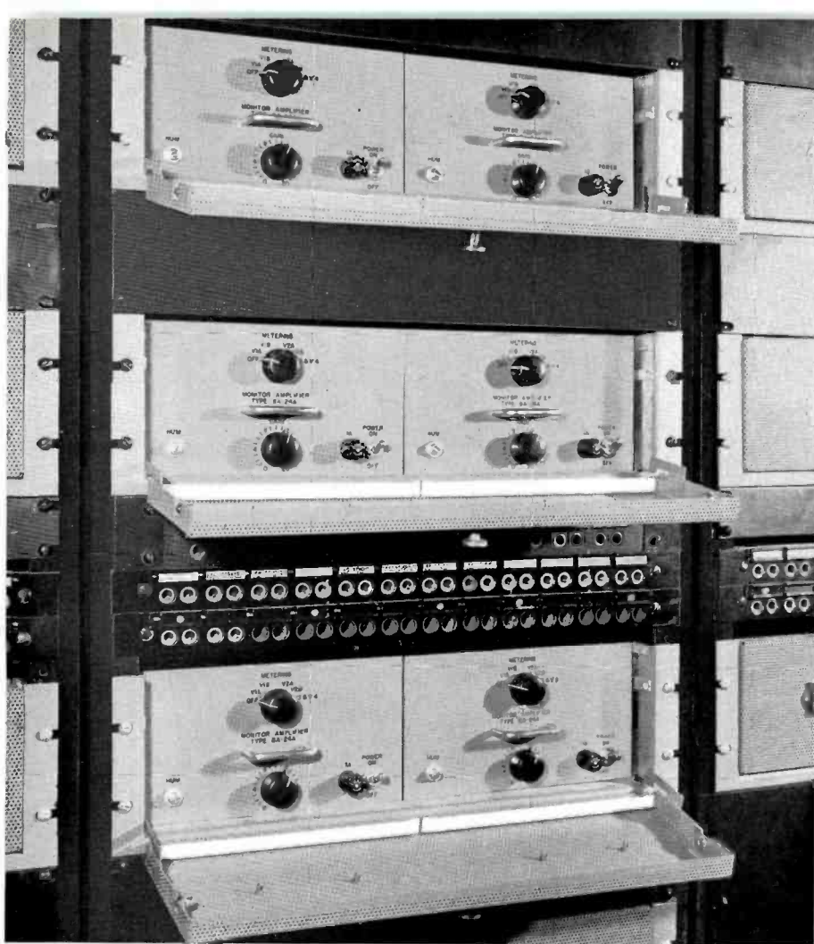
FIG. 6. View showing BA-24A Monitoring Amplifiers at NBC Studios in New York.
