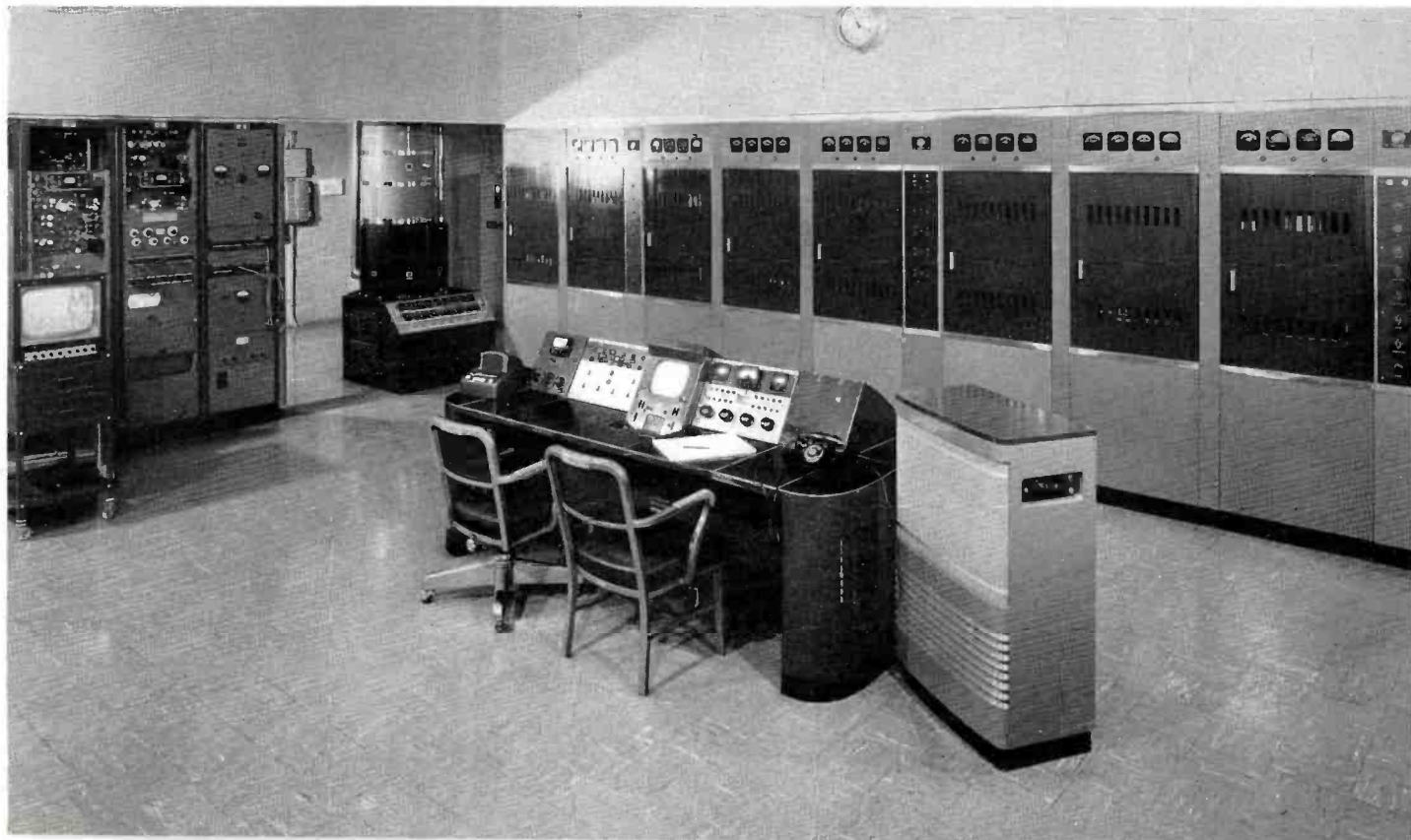
FIG. 12. WHIO's RCA TT-25BH Transmitter is the center of a U-shaped equipment layout. Left of the U consists of racks for input and test equipment. Right of the U will be formed by WHIO's original RCA TT-5A Transmitter which will be moved from studio building and used as an emergency unit.
